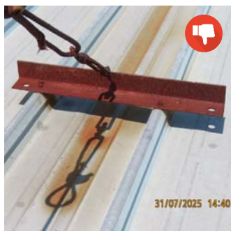
Galvanic corrosion can arise not only through direct contact, but also from water runoff or dripping from incompatible material
