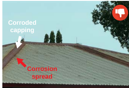
Mixing materials within the same roofing system may reduce the system's service life and increase the risk of premature corrosion
